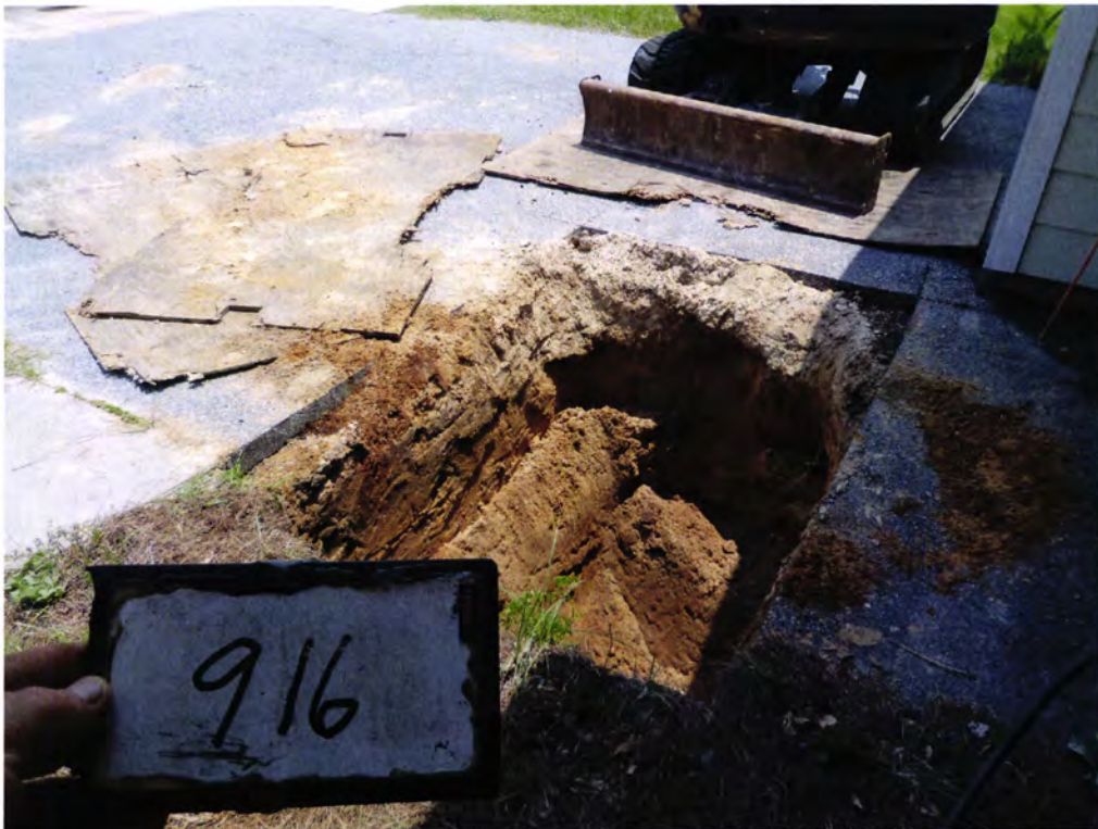
Picture 2: UST 916Barracuda excavation.
